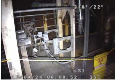
Examples of IPTZ camera LED lights illuminating BWR condenser bay areas at power - IPTZ cameras used in low light areas for leak detection
